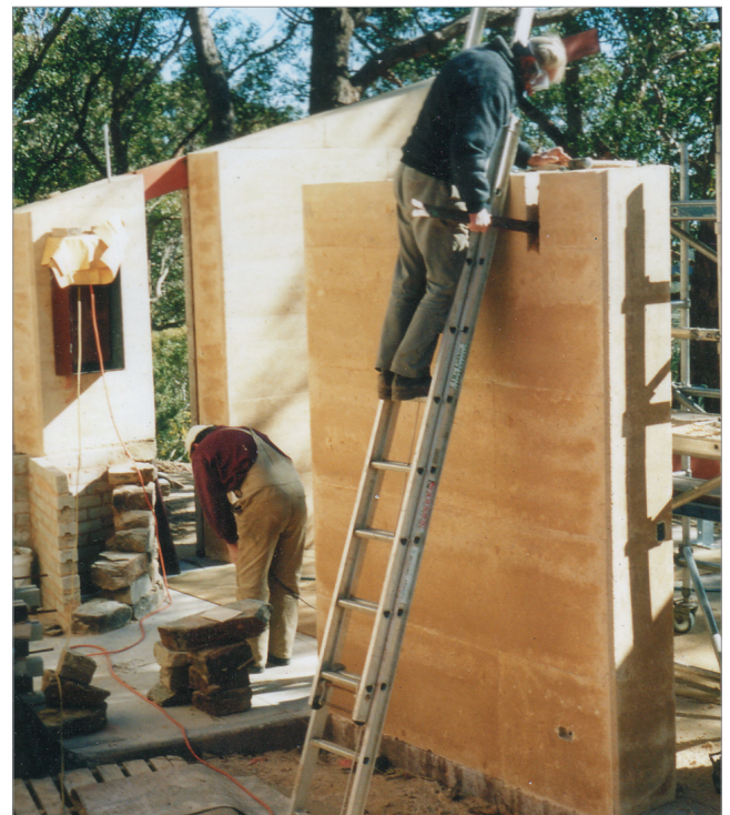
The rammed earth walls revealed.
